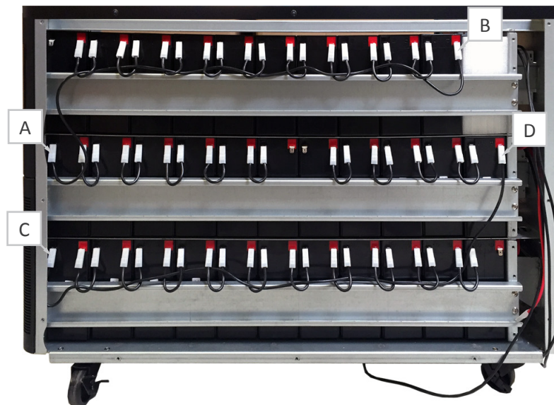
Front of Cabinet
