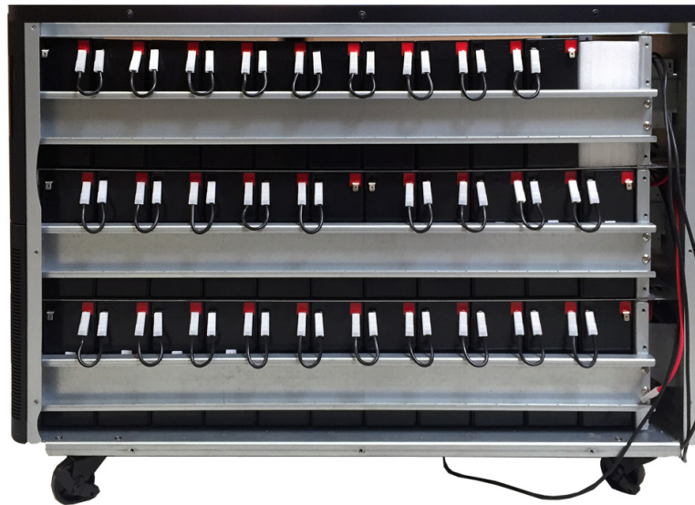
Front of Cabinet
