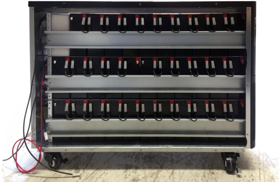
Rear of Cabinet
