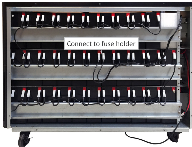
Front of Cabinet
