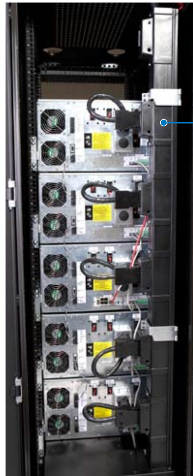
Powerware BladeUPS Parallel Bar
